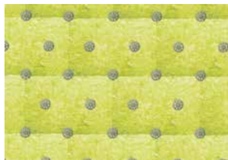
MINERAL WOOL – FIXINGS ARE PLACED CENTRALLY AND IN CORNERS OF NEIGHBOURING BOARDS
