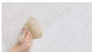
*optionally phase VI: When Pearl Patina dries, the surface can be coated with Decorative Varnish with addition of Brocade.
