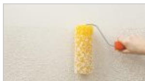
phase II: Apply Sandstone and form the texture with a sponge roller.
