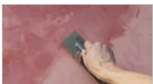
phase IV: Apply the third coat of Stucco, smooth the surface as much as possible.
