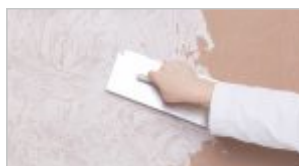
phase V: Apply light coloured Relief to fill gaps in the texture, smooth the surface.
