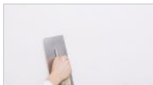
phase II: Apply approx. 2 mm thick coat of Relief with a venetian plastering trowel.
