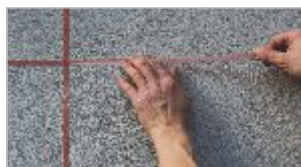
phase II: Apply tape imitating rustications when the Concrete surface dries.
