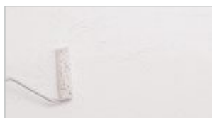
phase V: Apply coloured Pearl Patina with a roller upon the dry surface.
