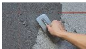
phase III: Moist the surface with water before application of the second Concrete coat, apply the material then.
