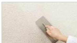
phase III: Smooth the drying material with a trowel edge.
