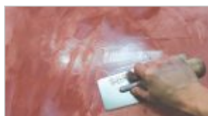
phase VI: Apply a coat of Decorative Wax and polish the surface.
