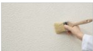
phase IV: Slightly grind with sandpaper and coat with Decorative Varnish.
