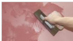
phase III: Apply the second coat of Stucco.
