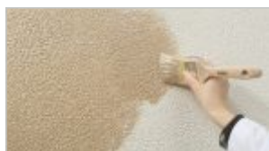
phase V: Apply coloured Pearl Patina with a paintbrush. Patina should be applied with irregular crossing moves led in all directions.
