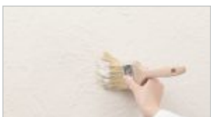
phase IV: Coat the surface with Decorative Varnish.
