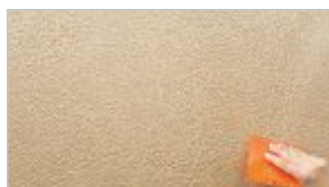
phase VI: Collect excessive material with a wall scraper.
