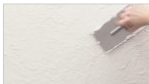
phase III: Shape the pattern with a trowel led flat upon the material.
