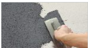
phase I: Apply Concrete upon the primed surface with a venetian plastering trowel.
