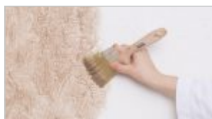
phase V: Apply Varnish coloured with Pigment.
