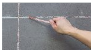
phase V: Remove previously applied tape as soon as the surface keeps moist.
