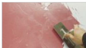
phase II: Apply the first thin coat of Classic Stucco, form the pattern simultaneously.
