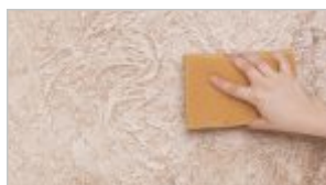
phase VI: Wash out excessive Varnish from material tops with a damp sponge.
