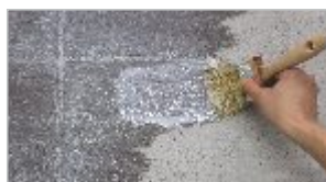
phase VI: Thoroughly coat the surface with Decorative Varnish.
