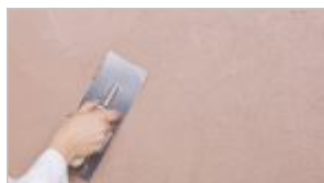
phase III: Form the pattern with a trowel applied flat upon the surface and dragged in various directions.
