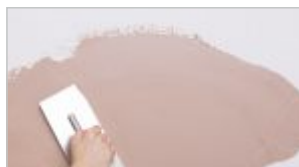
phase II: Apply approx. 2 mm thick coat of dark coloured Relief with a venetian plastering trowel.
