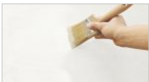
phase I: Prime the surface with Bonding Primer.
