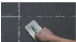
phase IV: When the material keeps drying, smooth the surface with a trowel edge until the expected level of smoothness is reached.
