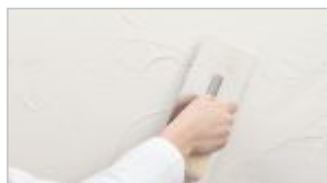
phase II: Apply approx. 2-3 mm thick uniform coat of Sandstone with a venetian plastering trowel.
