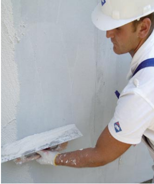
Applying renders using steel trowel
