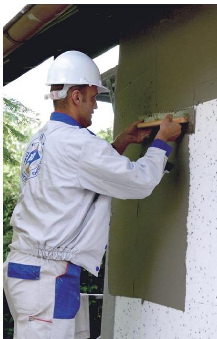
APPLICATION OF ADHESIVE ON POLYSTYRENE
