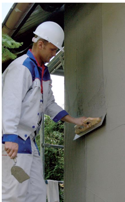
LEVELLING OF ADHESIVE WITH USE OF NOTCHED TROWEL
