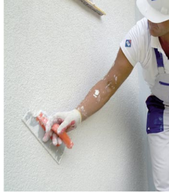
Applying renders using steel trowel
