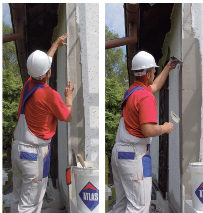
CORNER INSTALLATION
