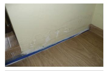
Photo 1. Dampness of floor area caused by the errors in the waterproofing execution
