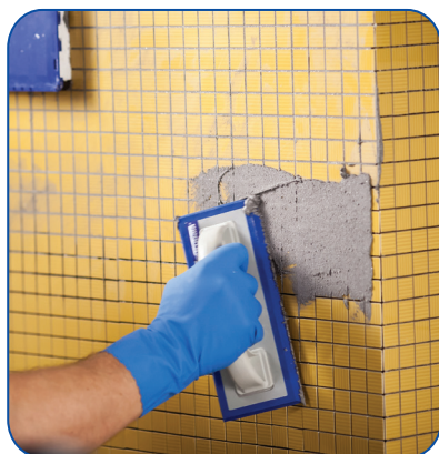
Photo 5. Decorative grout ATLAS/AVAL Artis Style (with glitter effect) perfectly matches with ceramic and glass mosaic. Glitter is present in the entire mass of the grout, therefore is clearly visible.
