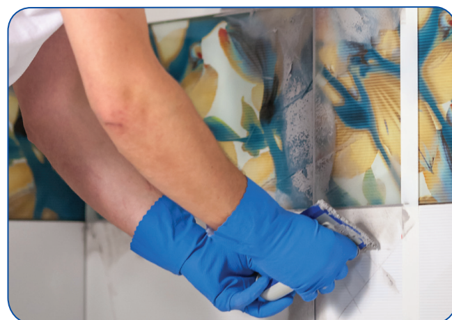
Photo 4. The float for grouting must be at an angle of approximately 45° and diagonally in relation to the direction of joints - this will ensure more accurate and easier filling. After filling the joints, one should wait until the initial mortar binding ends, which is when the grout becomes matt.
