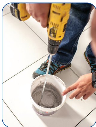
Photo 2. The cement mortar is prepared for use by mixing with water in the ratio listed on the packaging. Inadequate amount of water results in improper mortar setting - the mortar will not reach the intended technical and performance parameters, including the colour shade.
