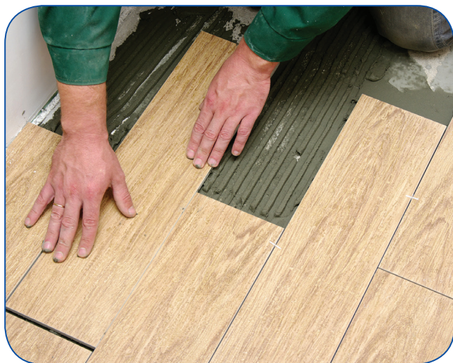
Photo 1. In offset arrangement, joints between the tiles are offset from each other by approx. 1/3 of the tile width - it's a common solution for the rectangular tiles. It is also possible to shift joints of about half of the tile width.
