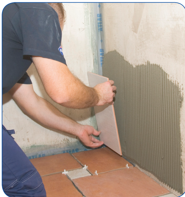
Photo 4. When the substrate is coated with damp proofing, the rules given by the membrane manufacturer should be followed. Usually, there are no contraindications for the use of C1 adhesives, but, due to the operational factors, it is advisable to choose C2 adhesives
