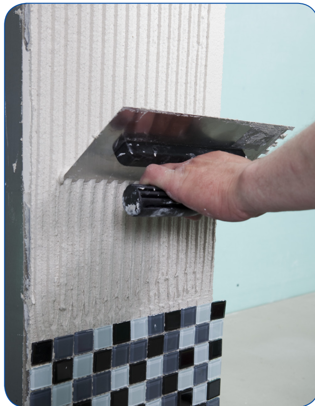
Photo 2. Too thick coat of an adhesive may cause immersing of mosaic tiles, flowing of mortar from the joints and the effect of corrugated surface, which will not form an ideal plane.
