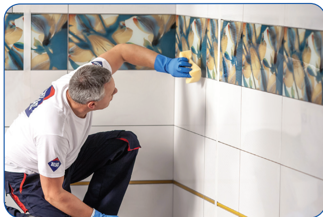
Photo 3. In case of epoxy grout one must wash joints and tiles with a cellulose sponge, soaked and well wrung, to remove visible dirt or dulling formed on the tiles surface. The final cleaning is carried out when the mortar hardens - after approx. 24 hours, one must wash the tiles with warm water with detergent or alcohol.
