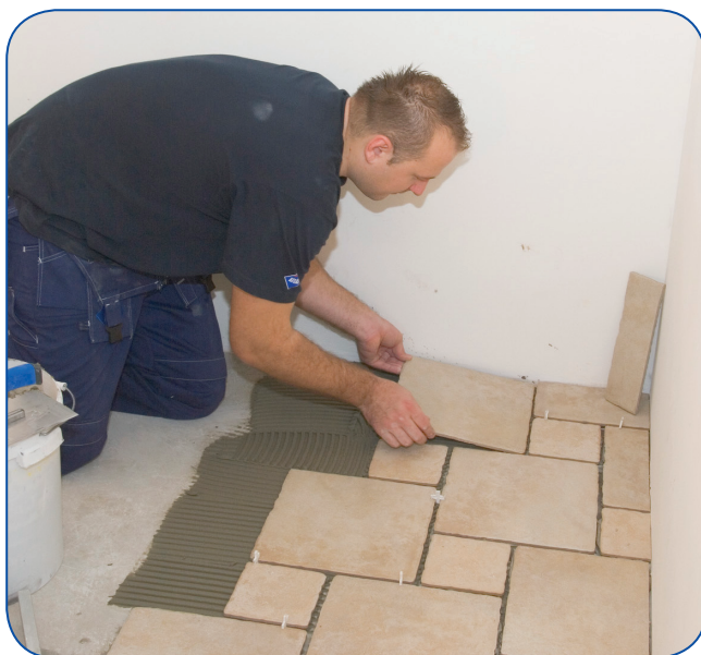
Photo 1. It is recommended to use the combined arrangement for the floor tiles fixing.
