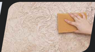
phase VI: Wash off excess of Varnish from material tops with a damp sponge.
