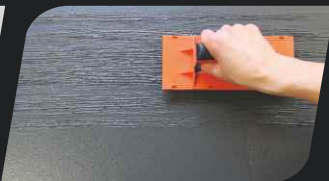
phase III: Shape the pattern by dragging the brush trowel upon the surface.
