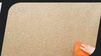
phase VI: Remove excess of material with a wall scraper.
