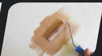
phase V: Apply coloured Pearl Patina with a roller with irregular crosswise moves led in all directions.
