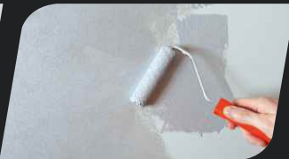
phase II: Apply the first coat of Diamonto with irregular moves of a string roller.
