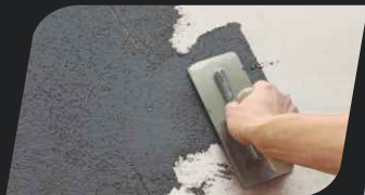
phase I: Apply the Concrete with a venetian trowel upon the surface previously primed with the Bonding Primer.
