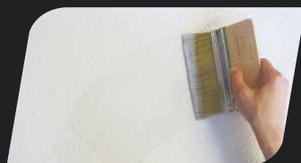
phase IV: Slightly treat the surface with a sanding paper, then cover it with colourless Decorative Varnish.
