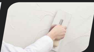
phase II: Apply 2-3 mm layer of Sandstone with a venetian trowel.
