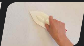
phase III: Smoothen the material with edge of trowel while the surface initially dries.
