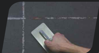
phase IV: While surface initially dries, smoothen it with an edge of trowel until obtaining desired level of smoothness.
