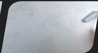
phase III: When the first coat dries, apply the second coat of Diamonto similarly to the previous one.
