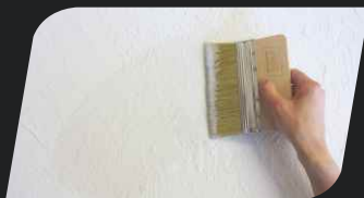
phase IV: Apply colourless Decorative Varnish upon the surface.
