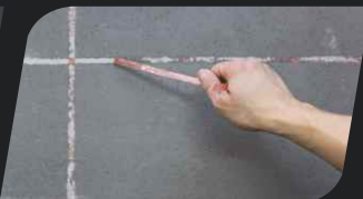
phase V: When surface is still wet, remove tapes.
