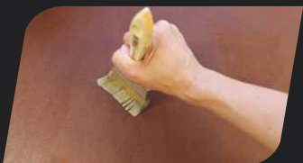
phase IV: After 24 h, apply colourless Decorative Varnish with a paintbrush or roller.
