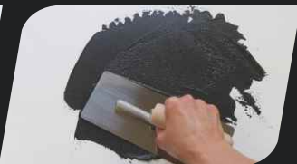
phase II: Apply coloured Sandstone with a venetian trowel.
