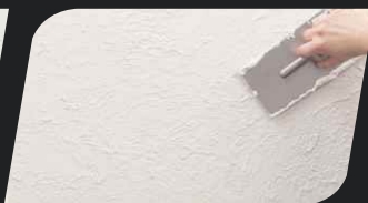
phase III: Shape the pattern with a trowel led flat upon the material.
