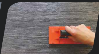
phase VI: While the surface is still wet, distribute DIAMENTO evenly with the brush trowel.
