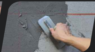
phase III: Slightly moisten the surface and apply a next layer of Concrete.
