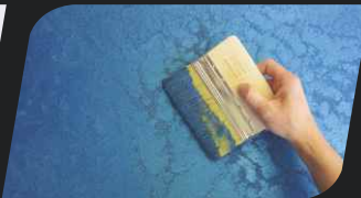
phase III: Start shaping the surface a few minutes after the paint application.
