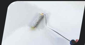
phase I: Apply base coat paint Initium Color upon clean and dry surface.
