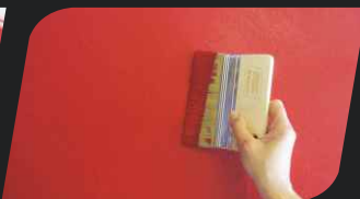
phase III: After a few minutes, start surface shaping.
