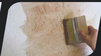
phase V: Apply Decorative Varnish coloured with the Pigment.
