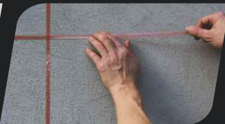
phase II: When the Concrete dries, adhere tape in order to imitate rustications.
