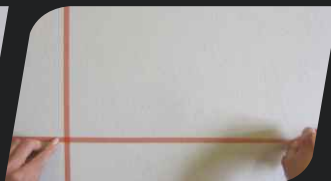
phase III: When the surface of Decorative Concrete initially dries, the tape which imitates rustications can be adhered.
