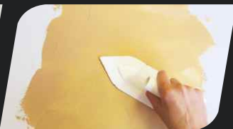
phase II: Apply layer of Pearl Relief with irregular moves of a plastic trowel in order to form the pattern.
