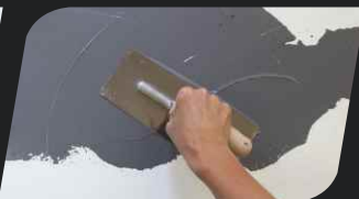
phase II: Apply a coat of Industrial Rust mixed with the Rust Activator.
