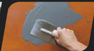
phase III: Apply the second coat in a similar way to the first one.
