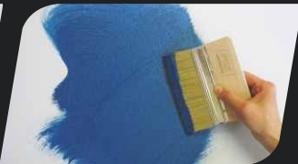
phase II: Apply coat of Diamento 3D with irregular moves of a paintbrush.
