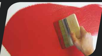
phase II: Apply coat of Kalahari Matt with an irregular moves of brush.
