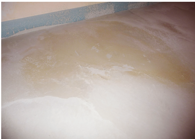
Photo 7. Appearance of surface executed with mortar containing too much water; anhydrite screed is not homogenous in colour – it is a result of the chemical additives elution
