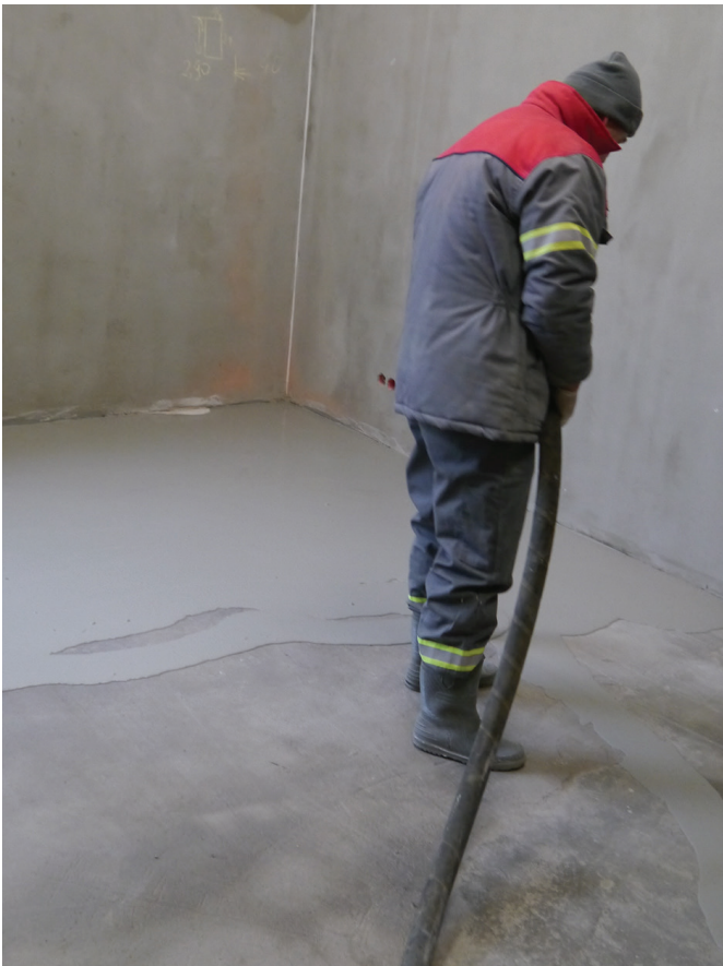
Photo 5. ATLAS SMS 15 and ATLAS SMS 30 self-leveling mortars can be mechanically applied on large surfaces.
