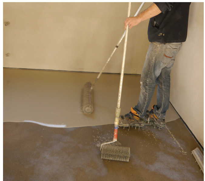
Photo 4. Unifying and de-aerating the mortar with a mesh roller.
