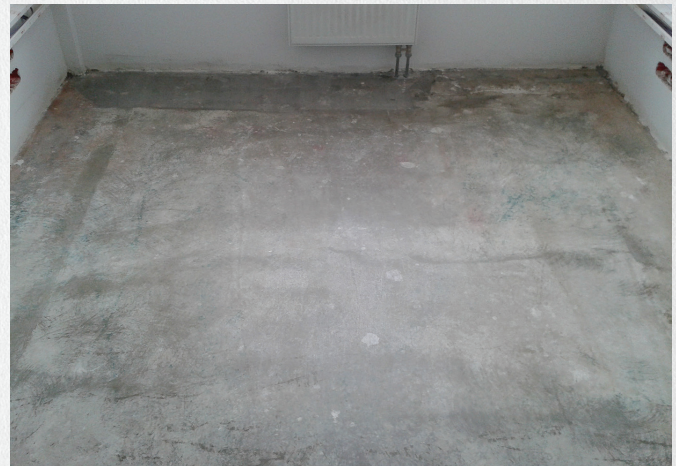
Photo 1. Priming with the use of ATLAS Uni-Grunt (AVAL KT 17) emulsion
