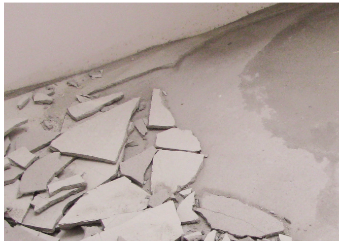
Photo 4. Loosening off the substrate
