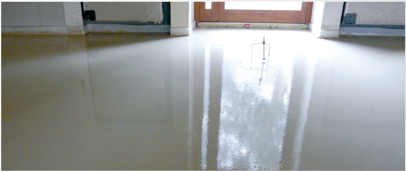
Photo 1. Machine application of the self-leveling screed on an old concrete substrate
