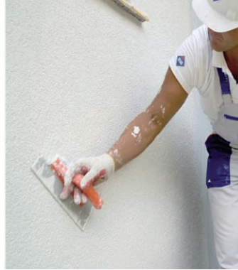
Applying renders using steel trowel
