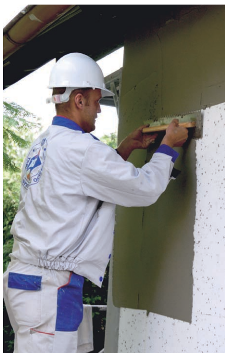
APPLICATION OF ADHESIVE ON POLYSTYRENE
