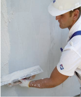
Applying renders using steel trowel
