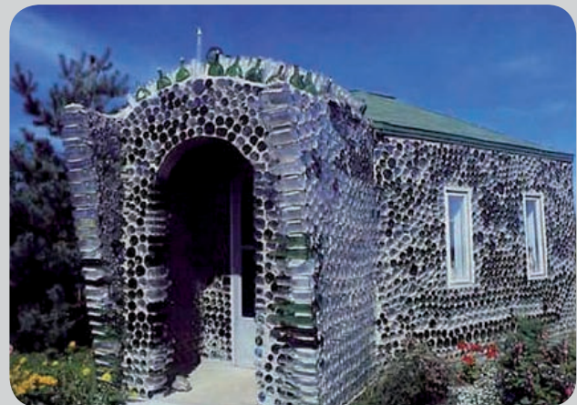
In the past, one way of the outer walls finishing was decorating the render with glass or stones.
