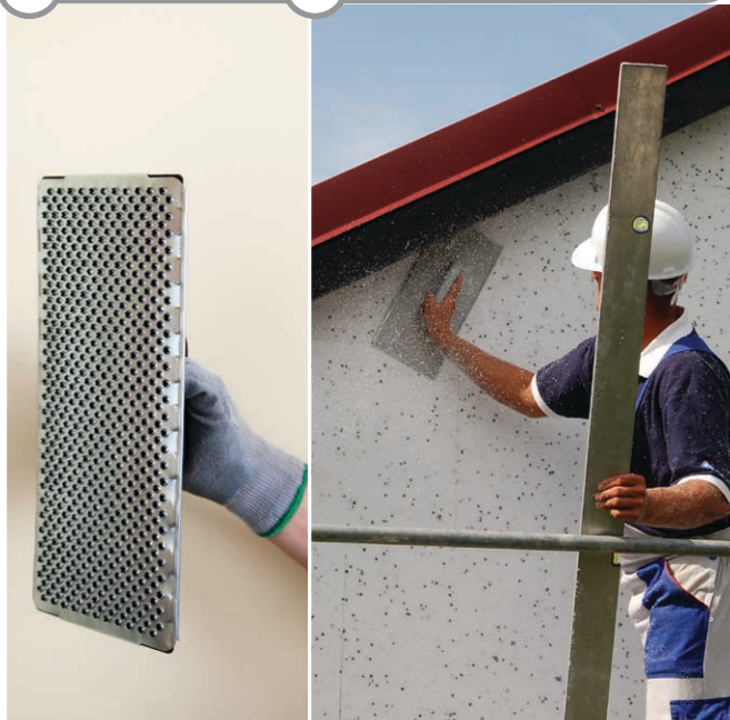
6 RASP | 6a PLANNING THE SURFACE WITH A RASP
