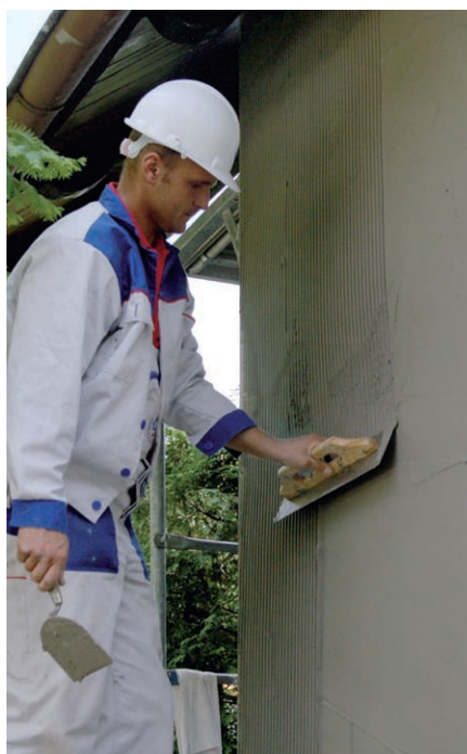
LEVELLING OF ADHESIVE WITH USE OF NOTCHED TROWEL
