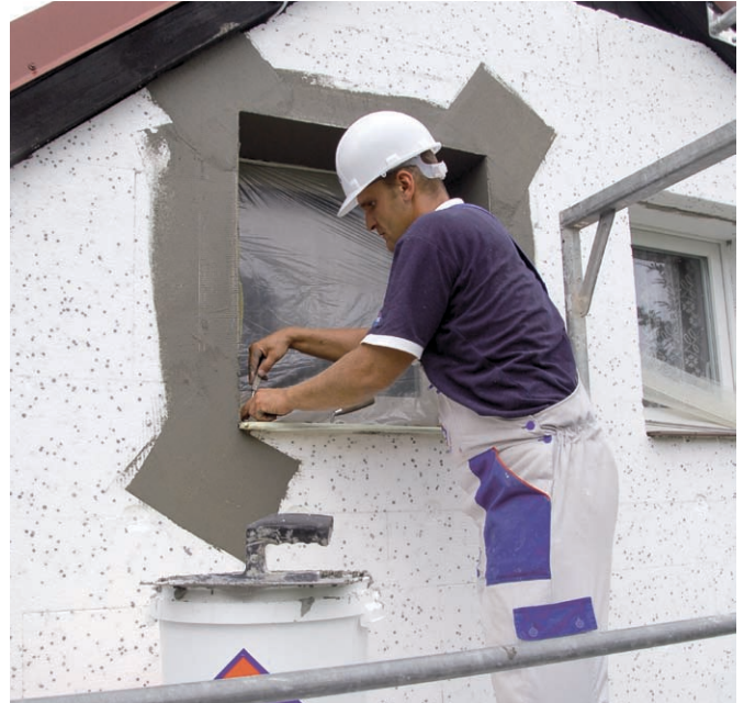
PREPARATION OF THE WINDOW REVEAL WITH THE USE OF CORNERS AND DIAGONALLY APPLIED MESH STRIPS
