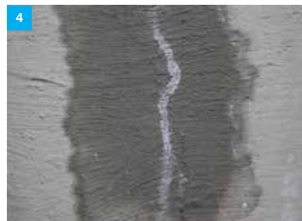
The crack is closed by salt crystals, no water seepage.
