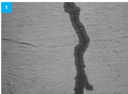
Active leak where the crack occurs in the substrate.
