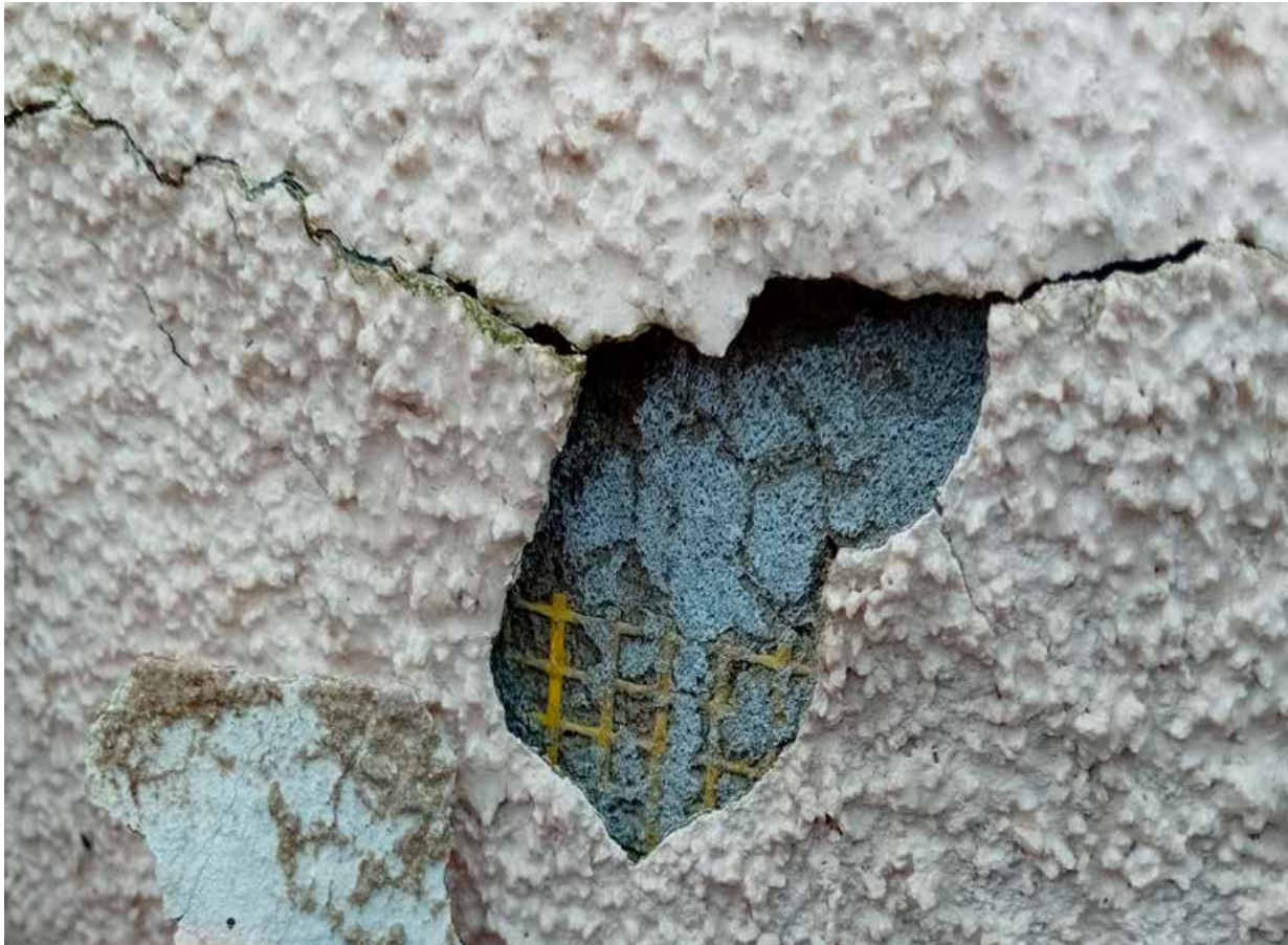
DAMAGED RENDER AND BASECOAT
