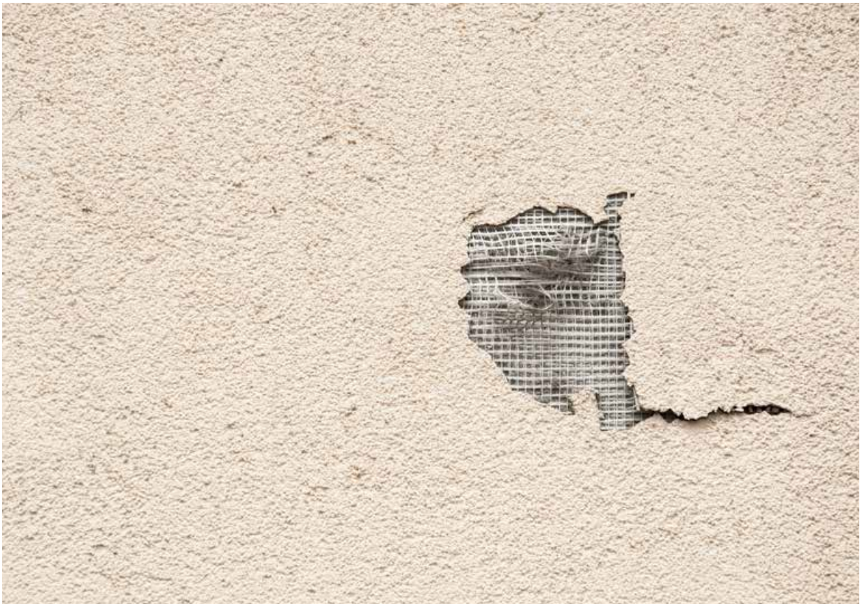
DAMAGED RENDER, BASECOAT AND THERMAL INSULATION
