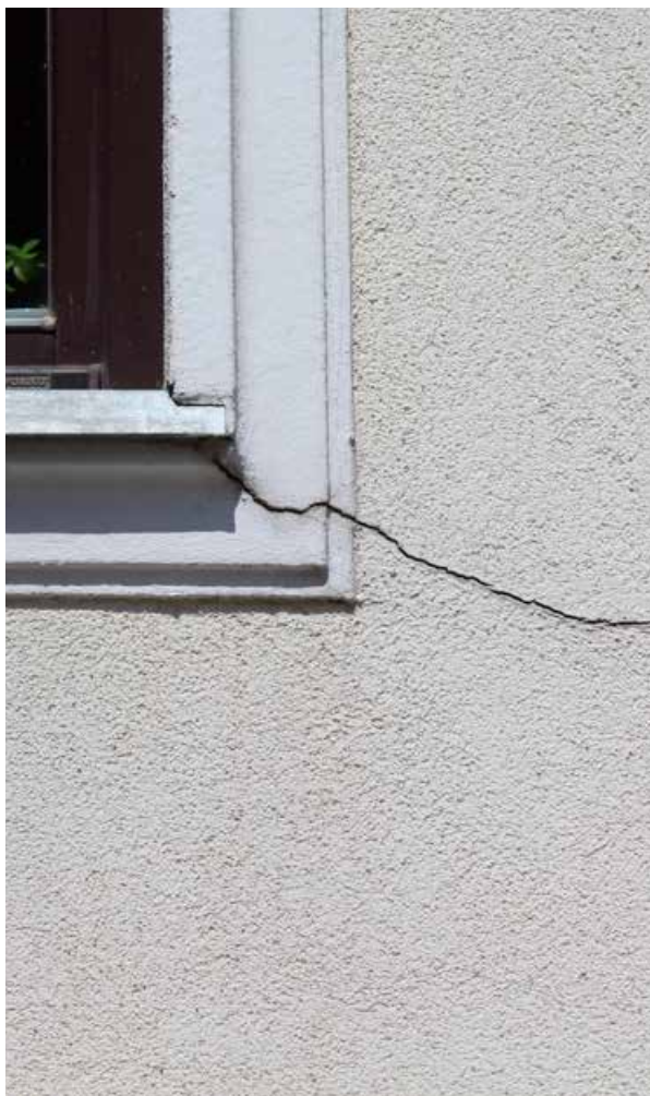
SINGLE CRACKS WIDER THAN 0.2 mm
