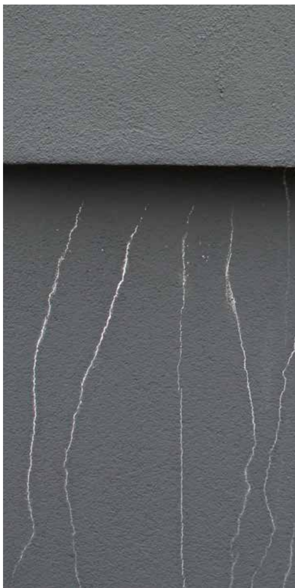
SALT EFFLORESCENCE, STREAKS, LIGHT SPOTS
