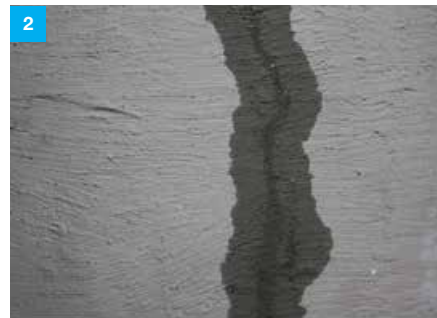
Gradual dampening of the insulating coating where the crack occurs.
