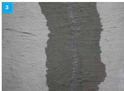
The crack is being gradually closed by crystallizing salts, there is still a slight water seepage. Effect after 7 days.
